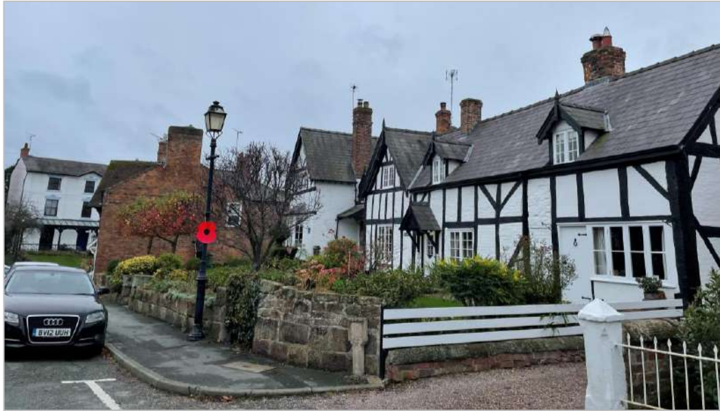
Figure 4.3: View south west of the grade II listed National Westminster Bank and house adjoining to the south (17 th century), showing the use of timber-framing within the TCA
