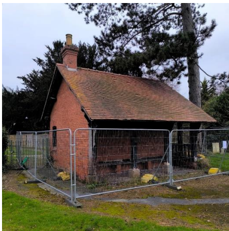
Fig. 1: Gardeners hut at Overleigh Cemetery (South)
