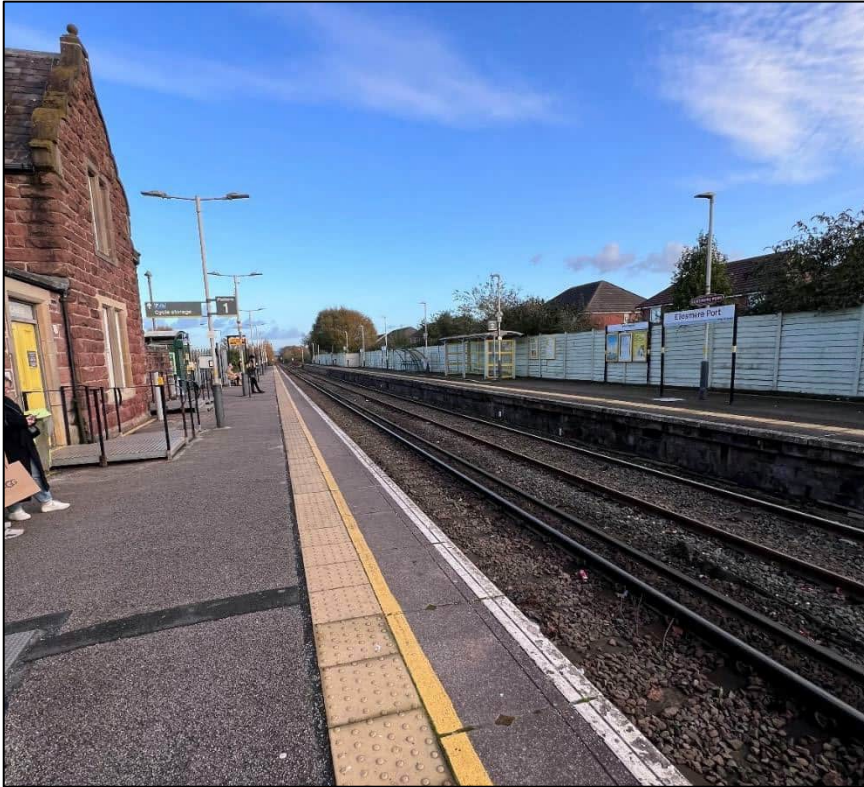
Figure 2-12: Ellesmere Port Railway Station
