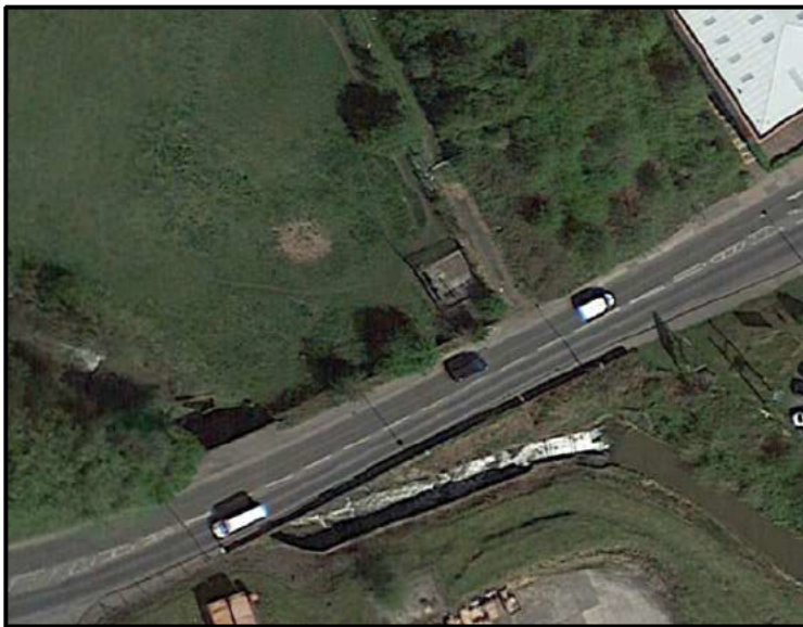
NORTH SOUTH AERIAL VIEW
